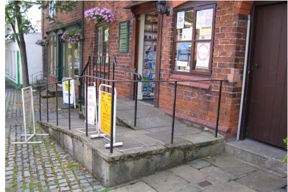
Pharmacy, The Cobbles - showing contemporary access ramps
