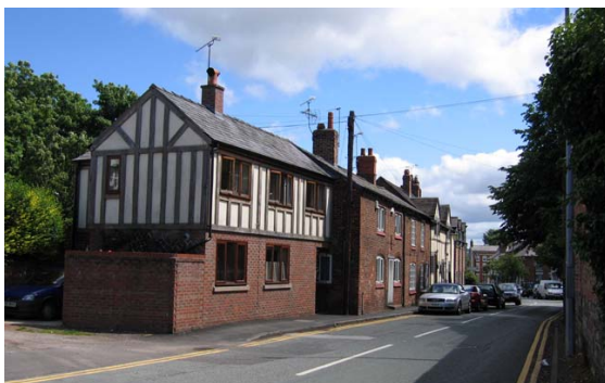
Modern timber framed building at 43 High Street
